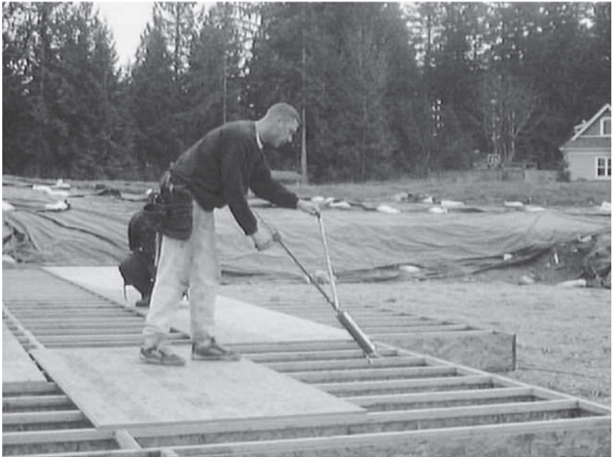
Figure 16-6. (A) Traditional method of applying glue to floor joists. (B) New method using commercially available extended gun ($50 retail). A handle was added to the gun to reduce hand/wrist fatigue (parts less than $10). Job times were the same for each of the two methods. (Photographs by Barbara Silverstein.)
