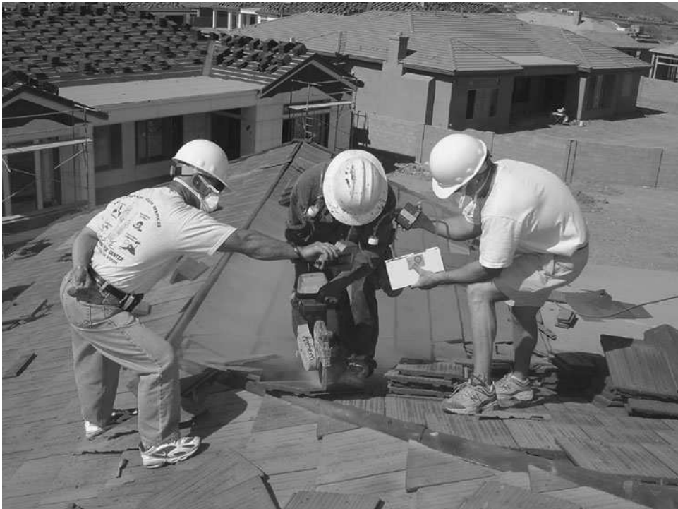
Figure 34-2. Industrial hygienists collect follow-up samples for a silica exposure among roofers. (Courtesy of the National Institute for Occupational Safety and Health.)
